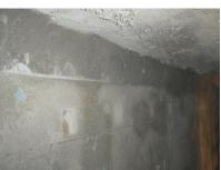
ULTRA TEK 70 NC Wall Cast with top section Shotcreted
