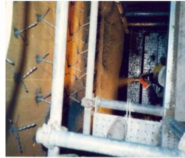
The low dust and rebounds result from the Ultra-Set advantage
