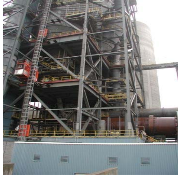
Cement Kiln Preheat Tower
