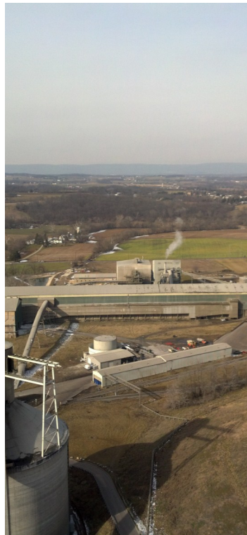
From the top of a cement preheat tower. Pretty high up there!
