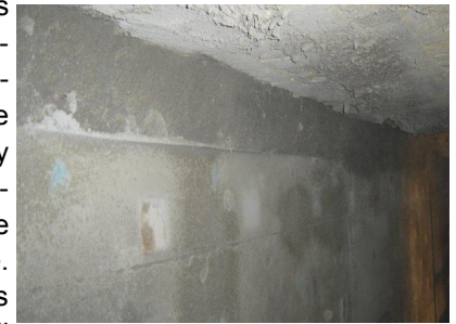
ULTRA TEK 70 NC Wall Cast with top section Shotcreted
