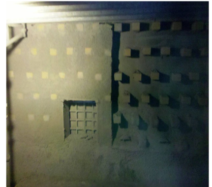
A gunned Q-TEK wall looks just like a rammed plastic wall, minus the laminations
