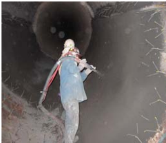
Shotcrete is being commonly used in lime and aggregate kilns
